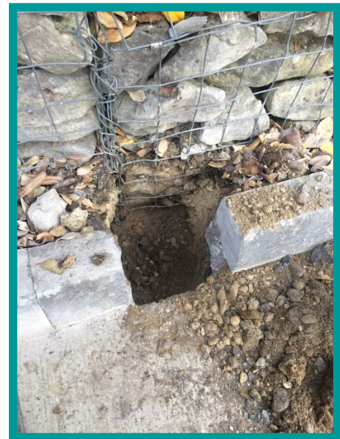
Foundations are dug
