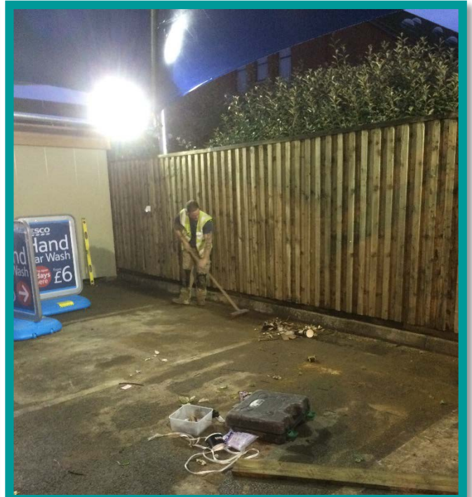
Cleaning up after completion
