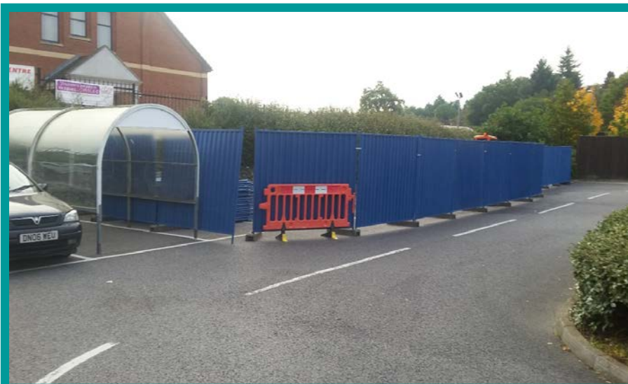
Area of installation is sealed off
