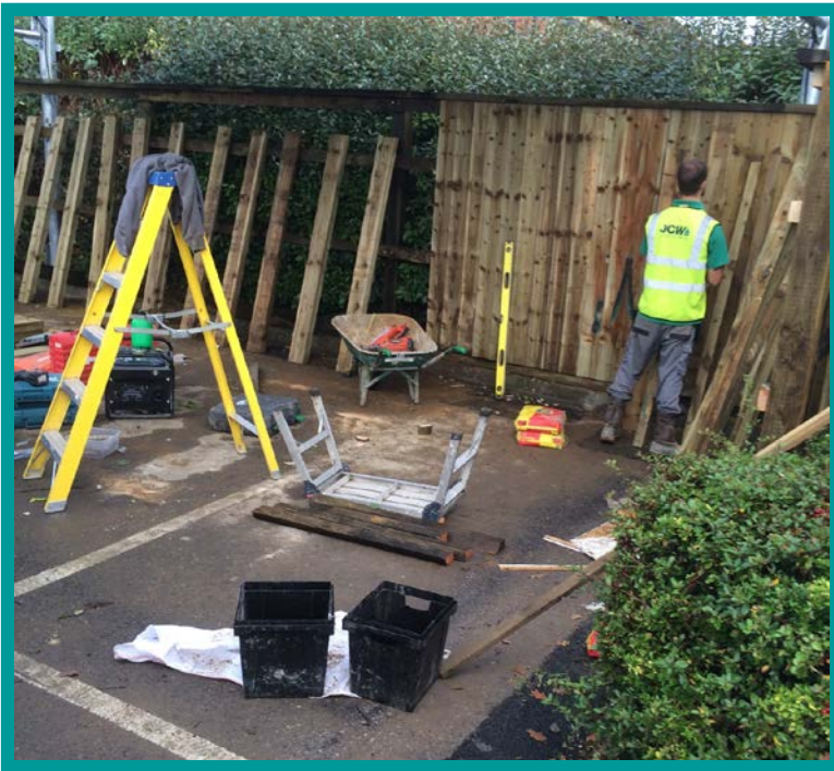
Erecting the fence
